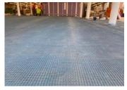
Schönox Renotex ® 3D was rolled in place, acting as a decoupling layer eliminating any issues with adherence to the plywood or insulation panels.
